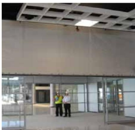
Fibershield V protecting an existing installation of non-fire rated glazing
