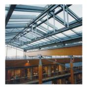
Ventria is a transparent natural ventilator and is also suitable for smoke and heat ventilation purposes.
