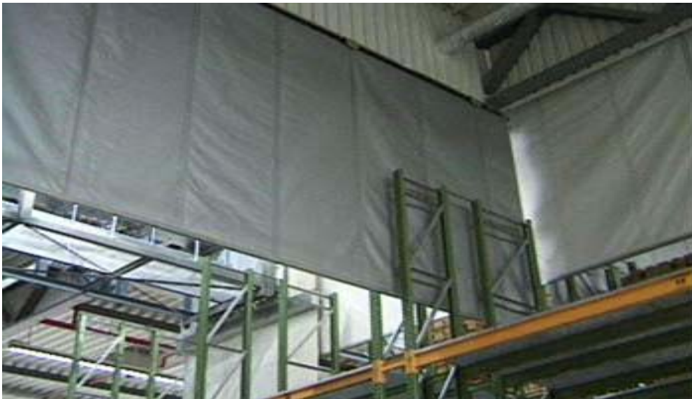
Figure 1.1: Typical SMOKEHALT FS Installation
