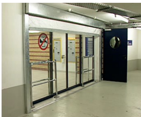
Fiberseal FS fire and smoke containment screen used to separate a car park from a shopping centre to upgrade existing glazing system. The system has commenced deployment.
